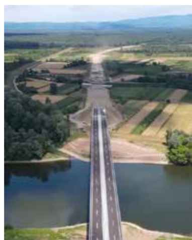
Gradiška Bridge completed: EU contributed with €3.2 million in grants August 2022
