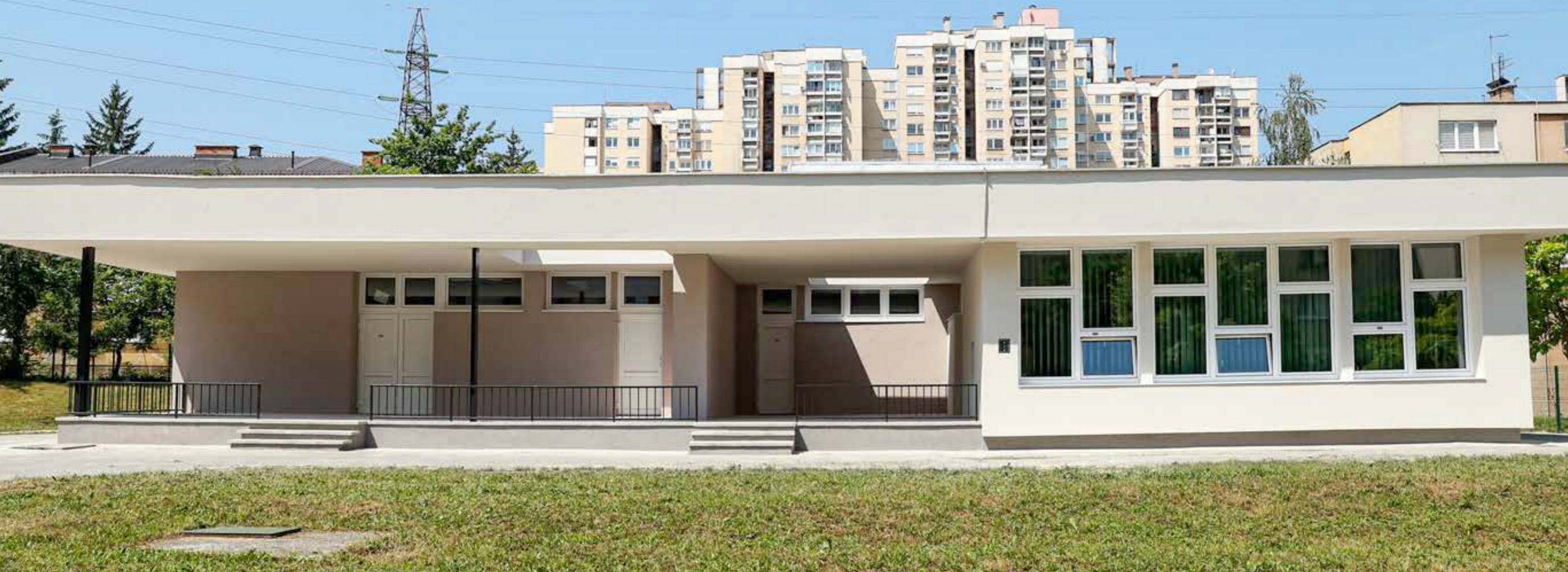
Kindergarten "Labudovi", Sarajevo, Bosnia and Herzegovina Regional Energy Efficiency Programme (REEP)
